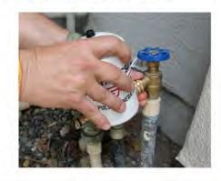
Connect the PG-2 at the spigot or water source: if on a swimming pool or other plumbing, plumb in a spigot for lines to be traced with a 3/4 inch MHT. Connect to inlet of the PG-2.
